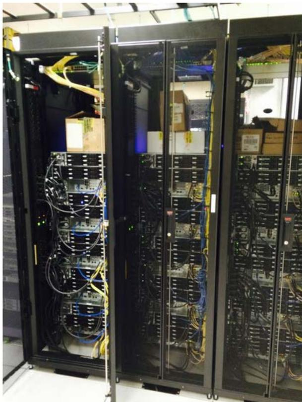
Figure 3: The PanSTARRS two-petabyte (2000-terabyte) storage array and its servers installed in the Institute's computing center.
